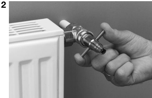
2 Unscrew the gland nut (water will not escape as the valve has an additional seal).
