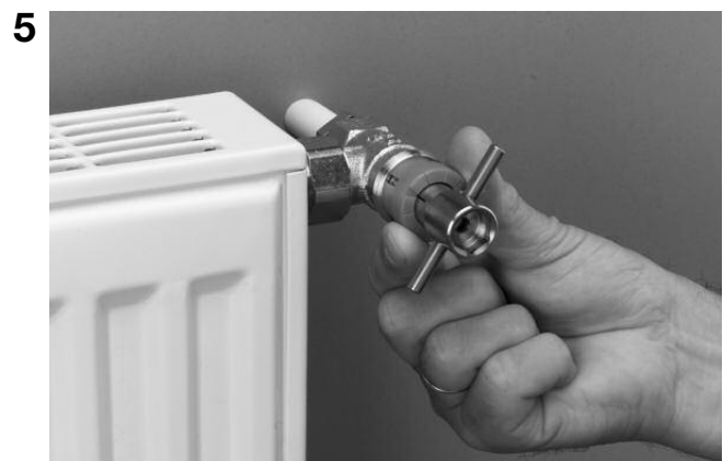
Bring the arrow on the setting ring in line with the marking on the presetting key.
