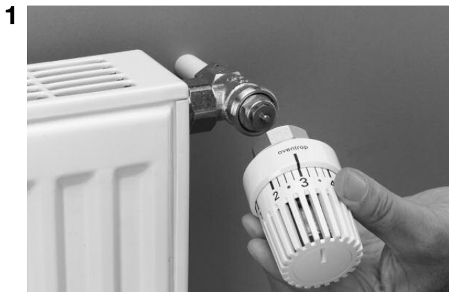
Unscrew the thermostat from the valve body.
