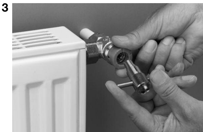
Place the setting ring onto the valve.
