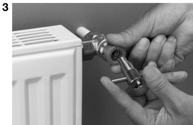
Place the setting ring onto the valve.
