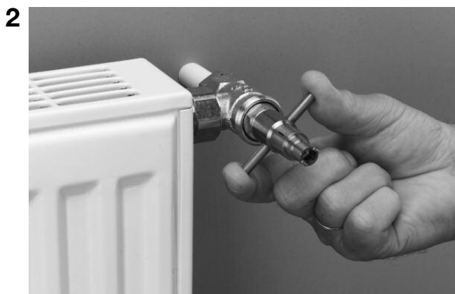
Unscrew the gland nut (water will not escape as the valve has an additional seal).
