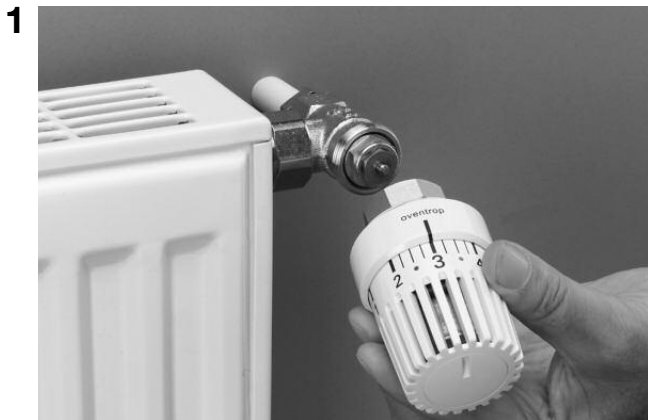
Unscrew the thermostat from the valve body.
