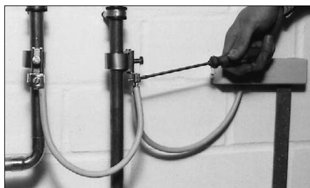
Illistr. 9: For equipotential bonding, fix earth clips onto both solar circuit pipes and connect a cable with a minimum section of 6 mm<sup>2</sup> to the main equipotential bonding rail.
