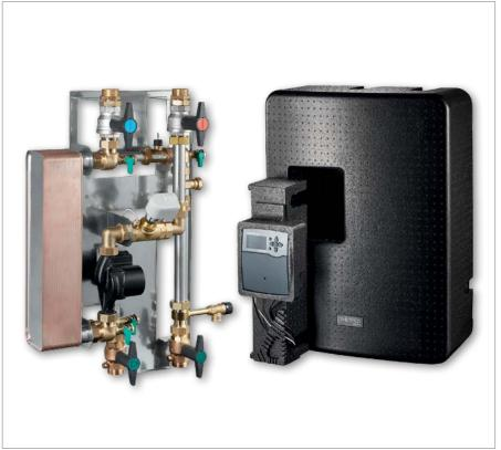
Station for hot potable water preparation "Regumaq X-80" with electronic controller "Regtronic RQ"
