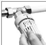
Photo 8: Replace handgrip loosely so that figure "3" is in line with the indicator mark.
