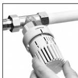
Photo 9: Turn handgrip to figure "2" while pressing it gently. Remove handgrip. (The calibration on the sensor casing is now turned to the right.)
