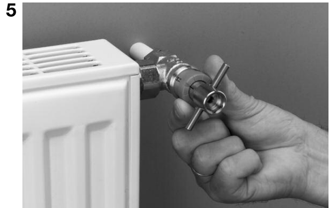
5 Bring the arrow on the setting ring in line with the marking on the presetting key.
