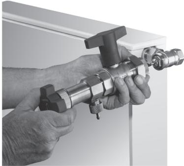
After having removed the thermostat from the valve, slightly loosen the valve insert with the help of a corresponding tool (M 30 x 1.5 spanner size 19 / M 30 x 1.0 spanner size 17). The “Demo-Bloc” is now screwed onto the valve.
