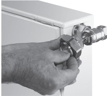
Where space is limited or where radiators are inside a casing, screw the attachment of the “Demo-Bloc” onto the valve first.
