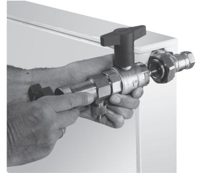
Screw the “Demo-Bloc” to the coupling.
