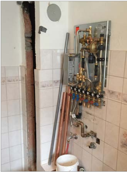
Installation of a “Regudis W” dwelling station
