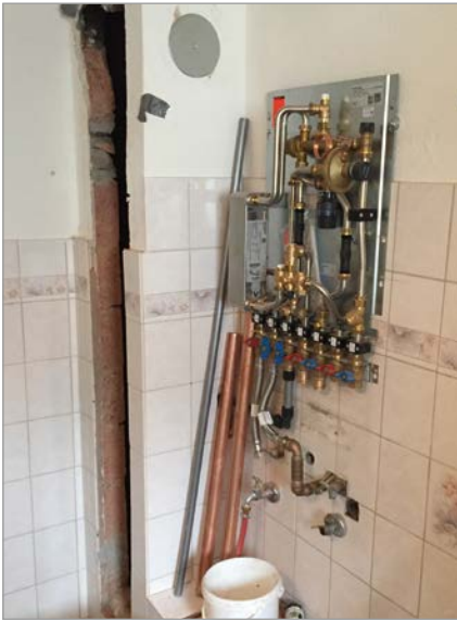
Installation of a “Regudis W” dwelling station
