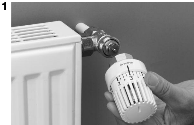
1 Unscrew the thermostat from the valve body.
