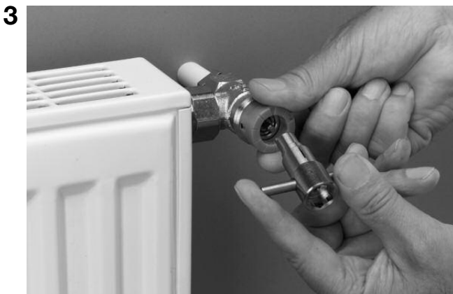
3 Place the setting ring onto the valve.
