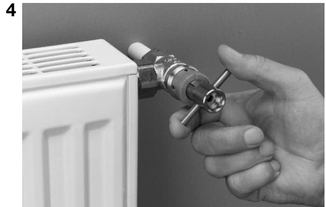
4 Close the presetting screw by turning the key clockwise until stop.
