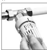
Photo 15: Replace handgrip so that figure "3" on the handgrip is in line with the indicator mark. Push down firmly with hand to secure.
