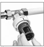
Photo 13: Remove handgrip. Turn sensor casing to the right until it is fully screwed into the body of the thermostat, then turn to the left again until the calibration mark (bore or white stroke) is in line with the indicator mark.
