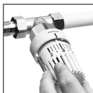
Photo 15: Replace handgrip so that figure "3" on the handgrip is in line with the indicator mark. Push down firmly with hand to secure.
