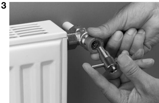
3 Place the setting ring onto the valve.
