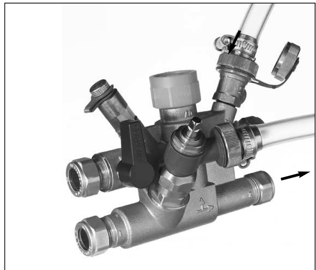
Illustr. 7 Flushing of isolated terminal unit
